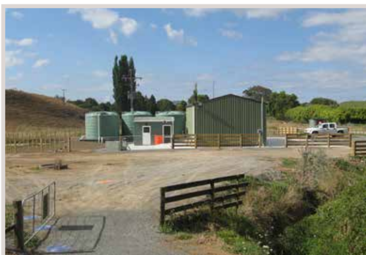
PIOPIO WATER TREATMENT PLANT
